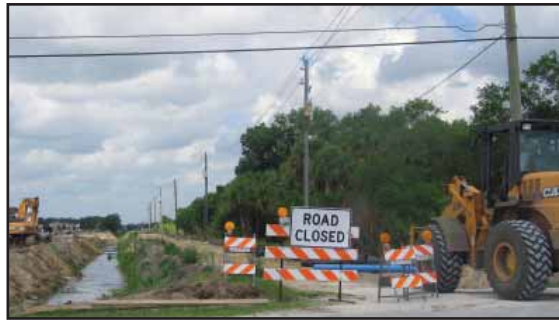
16th Street expansion project underway!
